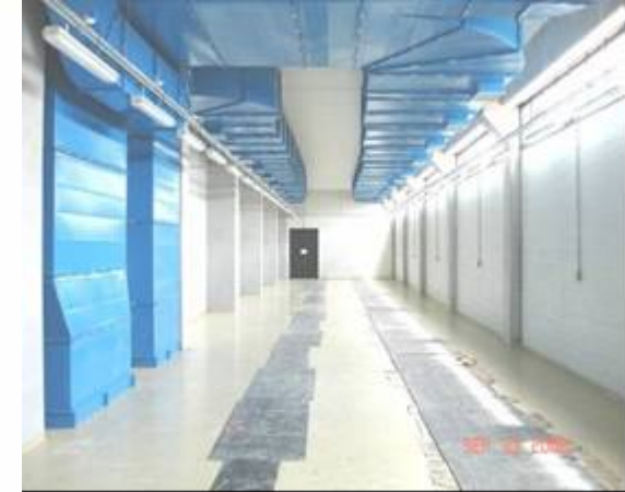
Turbo generator - Electricity room
