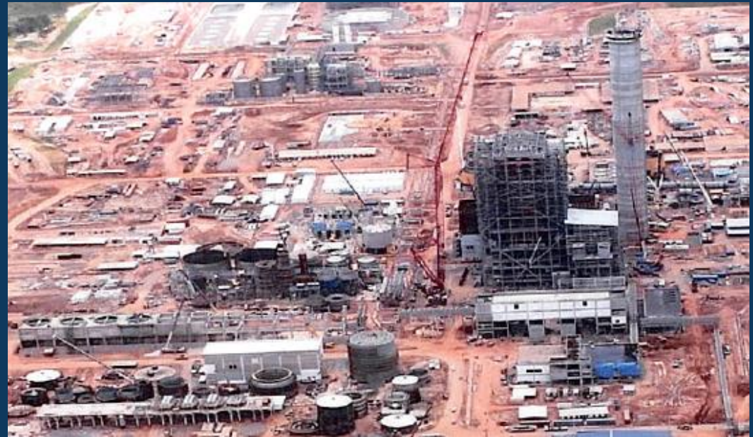
Panoramic View of Imperatriz Site - Maranhão Project
