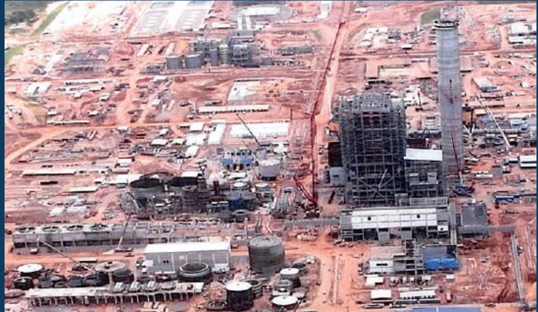
Panoramic View of Imperatriz Site - Maranhão Project
